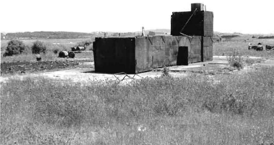
The foundations of the Pardoe factory in 1993. The concrete floor "built for all time" has so far lasted well. The metal structure has been added in recent times.
