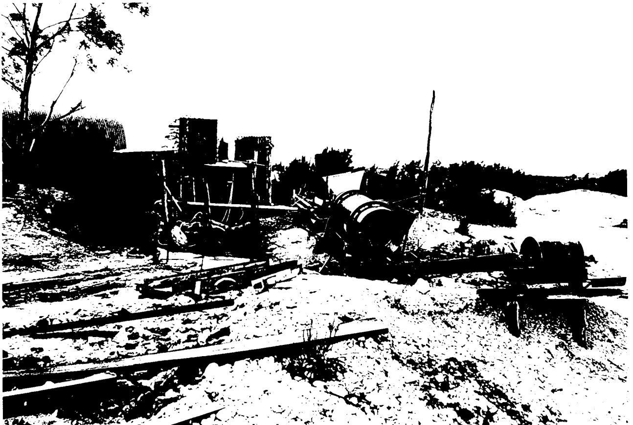
13. General view of processing area of mine site.
