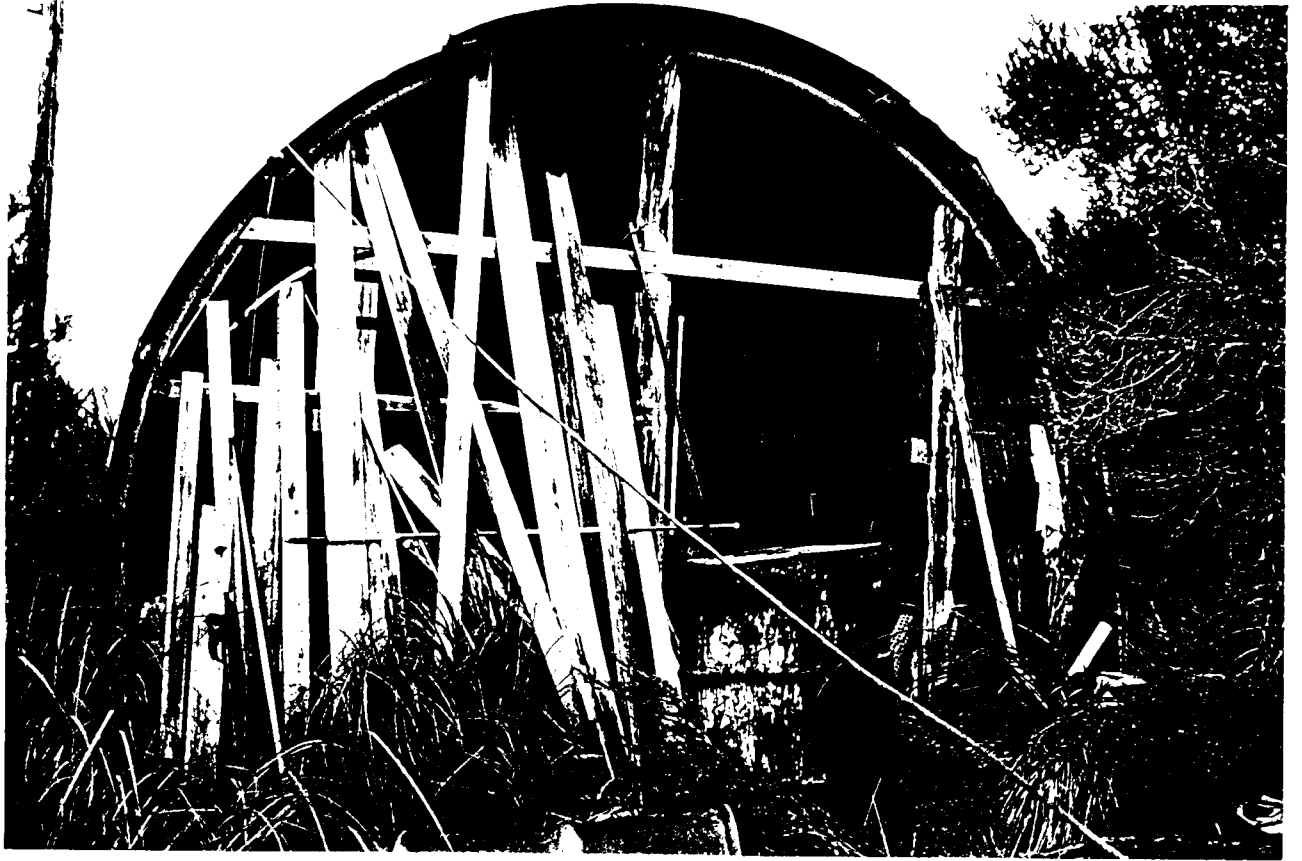
21. Southern Cross Shed - northern aspect.
